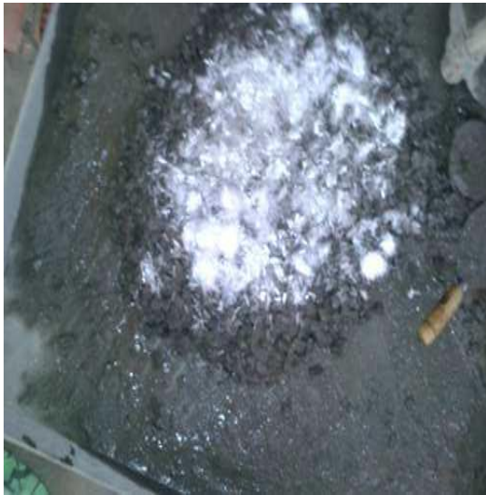
Fig 2 Mixing polypropylene fibers with concrete
