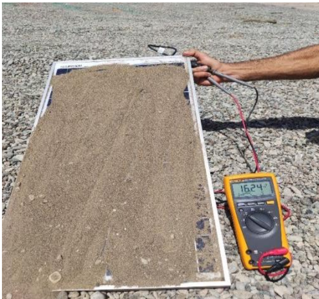
Fig. 5 Solar panel voltage with full of dust
