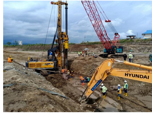
Fig 10:- Secant Pile Foundation Drill Tool Source: Author, (2021)
