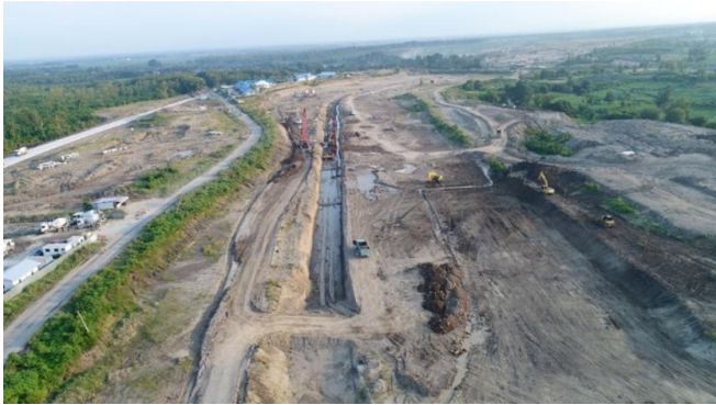
Fig 7:- Sectant Pile Foundation Work Area Source: Bendungan Semantok, (2021)
