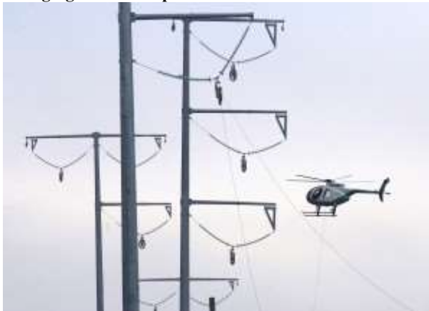
A helicopter starts the process of stringing a high-voltage transmission line
