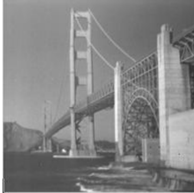
(a) Bridge image
