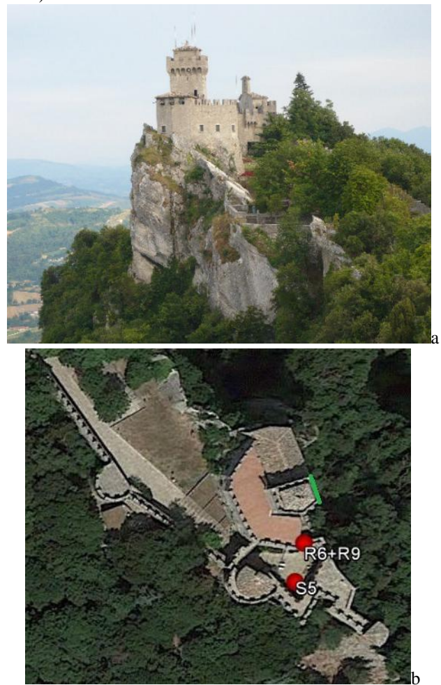
Fig. 4. Cesta Tower (a) and location of the measurements performed outside the building (b). The green line indicates the direction of the walls assumed as reference (N-S direction)
