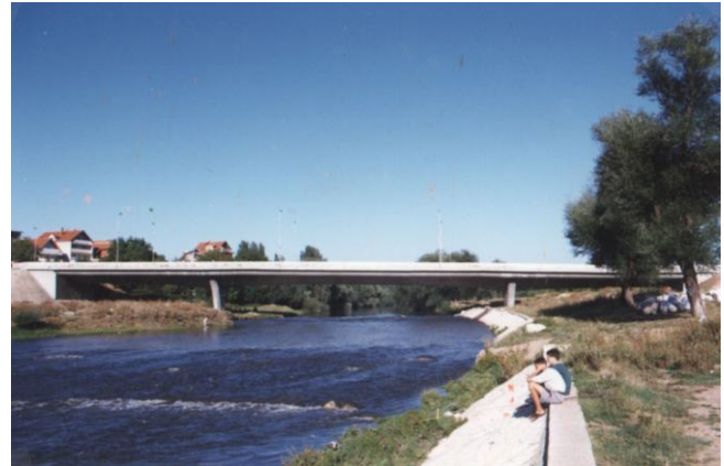
Fig.1 Photo of the road bridge over the Nišava
