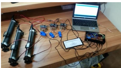
Figure 8. Testing of current and temperature monitoring system tools on an Internet of Things (IoT) -based distribution transformer.
