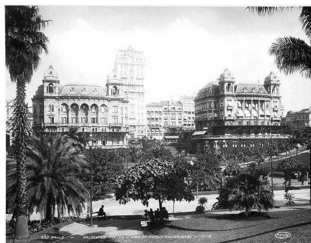
Fig. 2: The Prates buildings facing Anhangabau Valley in a photograph of 1930 [16].
