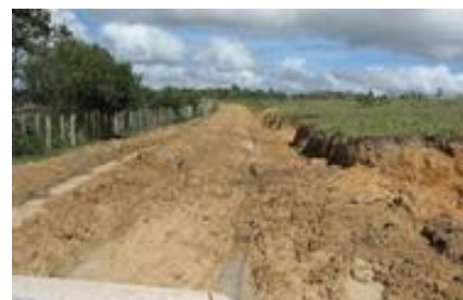
Fig. 7: Poor road conditions [21]
